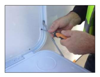
Please note that the silicone/sealant is not only for waterproofing the installation holes. It will also add strength. In most cases you will not screw the picnic table frame into a wall stud, therefore it is vital to use adequate, appropriate silicone/sealant.
